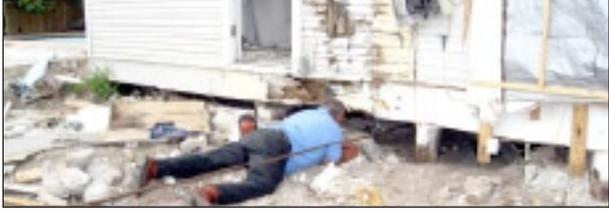
Below, the fireplace is taken off. Cutting off the bedroom and bathroom begins, then a beam is placed underneath during the separation.
