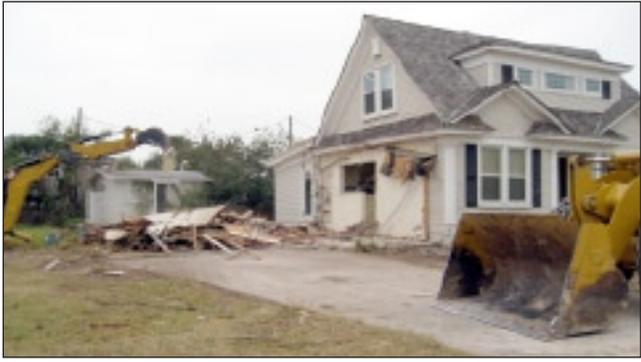
Above and below, workers demolish garage and breezeway of the Mercer house, and the materials go in the trash. Mr. Lara helps run rod under house as they start the preparations to remove the back portion.
